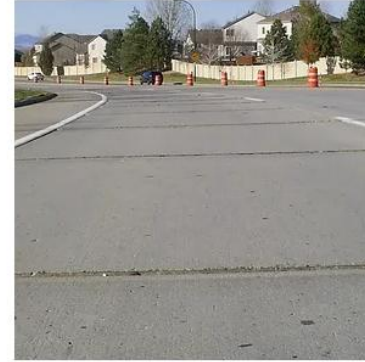
Faulted Joints
