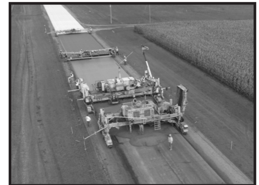
A drone's eye view of concrete paving on Cottonwood CSAH 1
