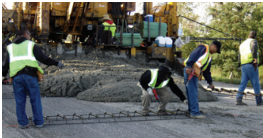
A crew from Manatt’s places a concrete overlay on U.S. 71 in Montgomery County, Iowa.
