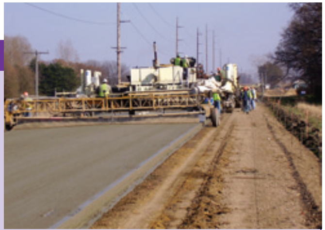
This concrete overlay was placed over a reclaimed asphalt base in Freeborn County, Minnesota.
