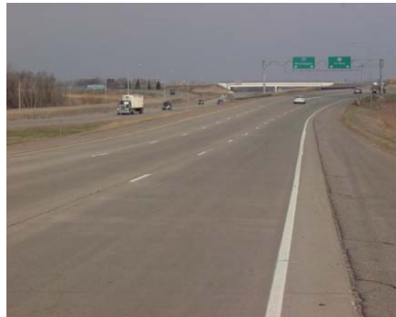
TH 55 concrete pavement in good condition.
