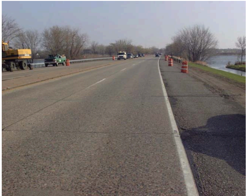
U.S. 61 Concrete Pavement— looking good after nearly 50 years!
