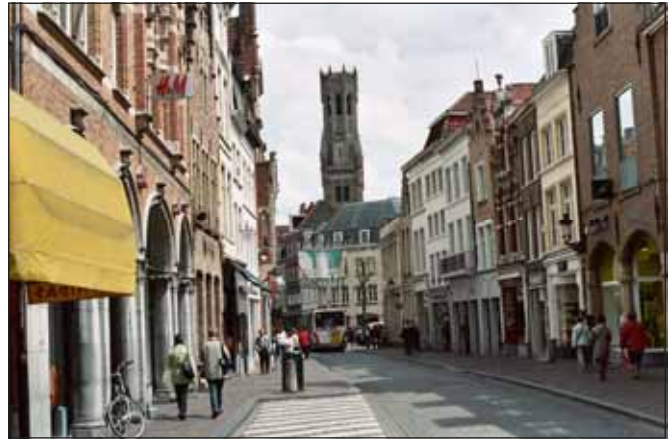
Typical street scene in Brugge, Belgium. Apparently, there is no incentive for smooth ride, nor are there any concerns regarding noise. Notice the cobblestone. However, the pavement is quite durable and has lasted for years.
