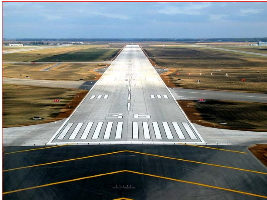
Newly constructed runway 18-36 at Hector Int'l Airport in Fargo
