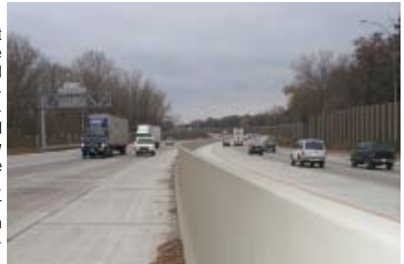
I-35W High-Performance "60-Year" PCC Pavement
